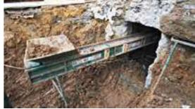
The Easikit<sup>™</sup> 450 is a simple and compact modular system with a large capacity, which is perfect for low volume material handling. Its robust design supports the removal of rubble and light hard core and it also has a detachable feed hopper.
